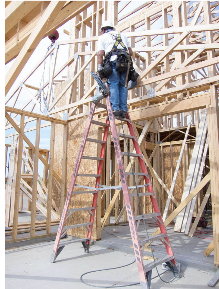
Worker using a personal fall arrest system on a ladder when using a tool that prevents 3 points of contact.
